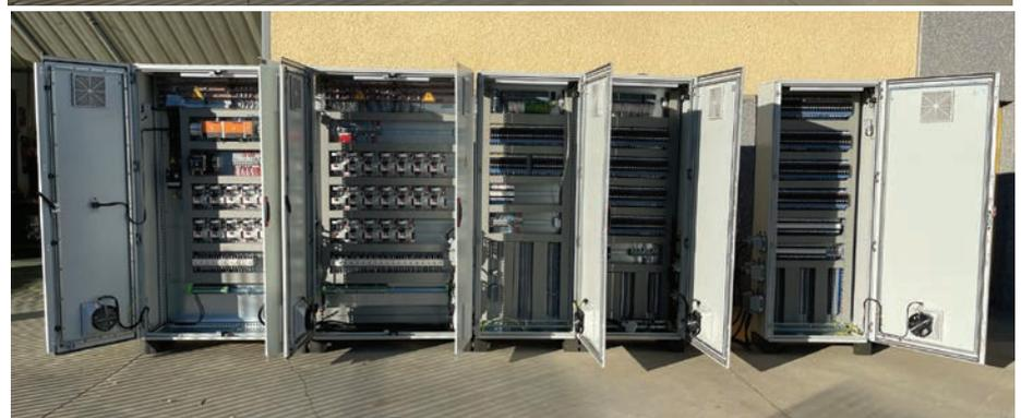
capacity is divided over two doors. With an IP55 protection degree, which protects against dust ingress that could be harmful for the normal operation, components inside the enclosure are well protected.
