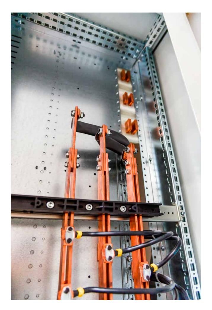
The design of floor standing enclosures within the nVent HOFFMAN Power System range, referred to as EPS, is based on the existing mild steel floor standing enclosure MKS and MCS, and allows for building Power Distribution and Automation Control panels.
