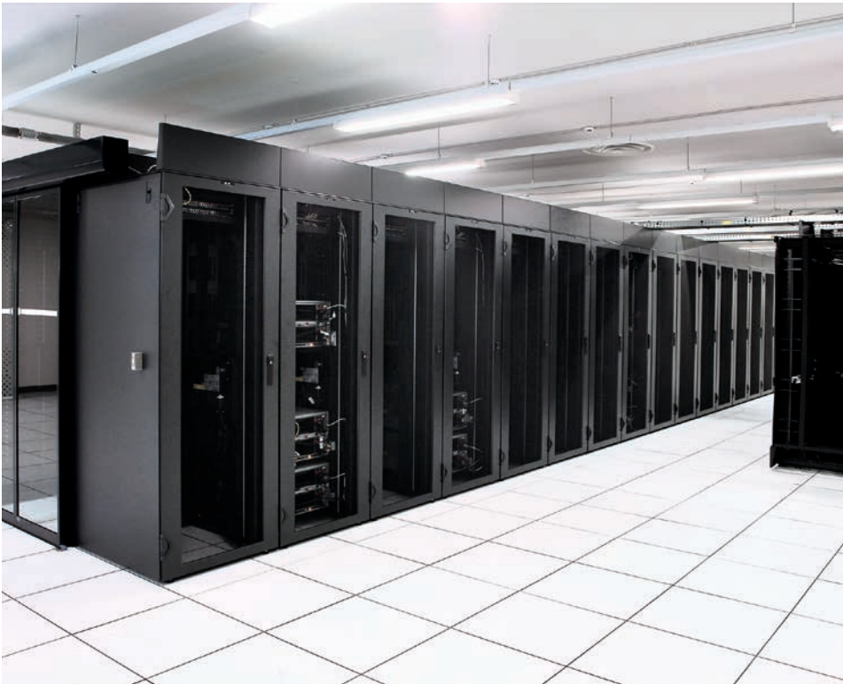
Hot-Aisle Containment
