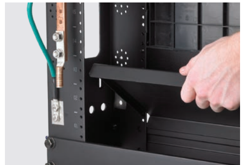
Bonding and grounding ready
