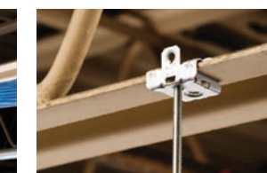
Threaded rod/chain/wire from beam
