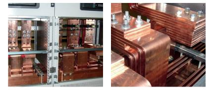
Using as a reference design the assemblies tested by Intertek-Semko, nVent HOFFMAN has created the design tables for the different busbar supports. Following the rules in this tables our customers can design derivations which will comply with the standard and making possible a short-circuit verification by comparison with a reference design using calculation. The design tables are included in Annex 04.
