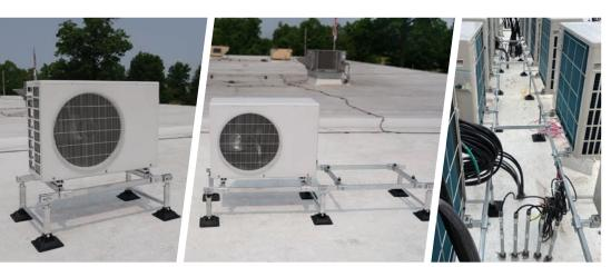
The nVent CADDY Pyramid Light-Duty Equipment Support is a fast, flexible and innovative system for supporting HVAC units on rooftop surfaces. Superior load distribution and a low abrasion foam interface combine to ensure that the roof membrane is protected despite varying roof surfaces and shifting caused by expansion and contraction.
