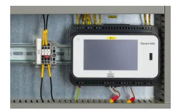
Next generation **DIN-mounted touch screen** heat tracing controller for **dual independent heating zone** control.
