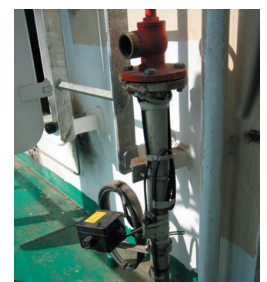
Pipe freeze protection for fire suppression
