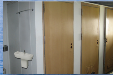
LIVING QUARTERS ■ Hot Water Temperature Maintenance ■ Floor Heating
