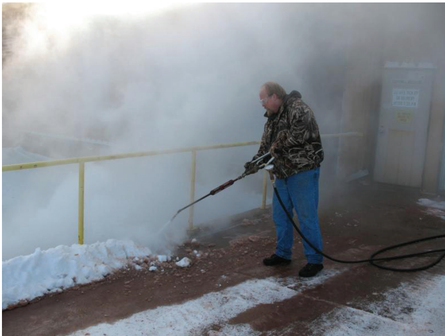
Figure 9. Ice removal using steam wands.
