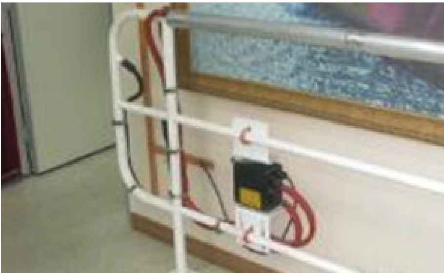
Figure 13. Heated Handrails
