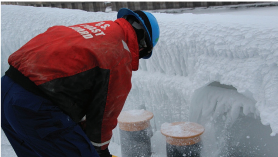
Figure 10. Ice removal using mechanical methods.
