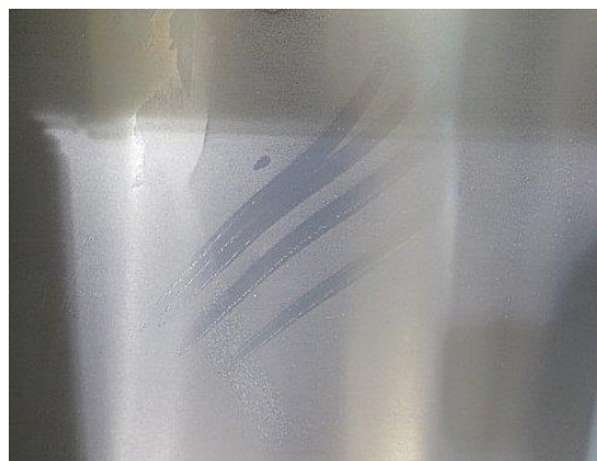
Condensation inside the cabinet
