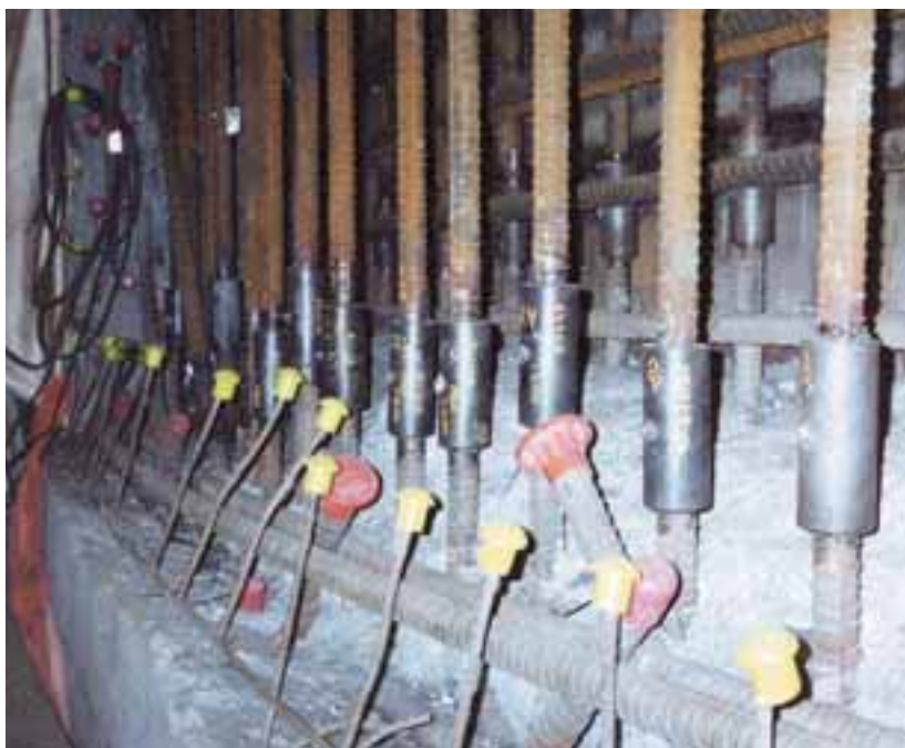
Steam Generator Change Out - Nuclear Power Plant
