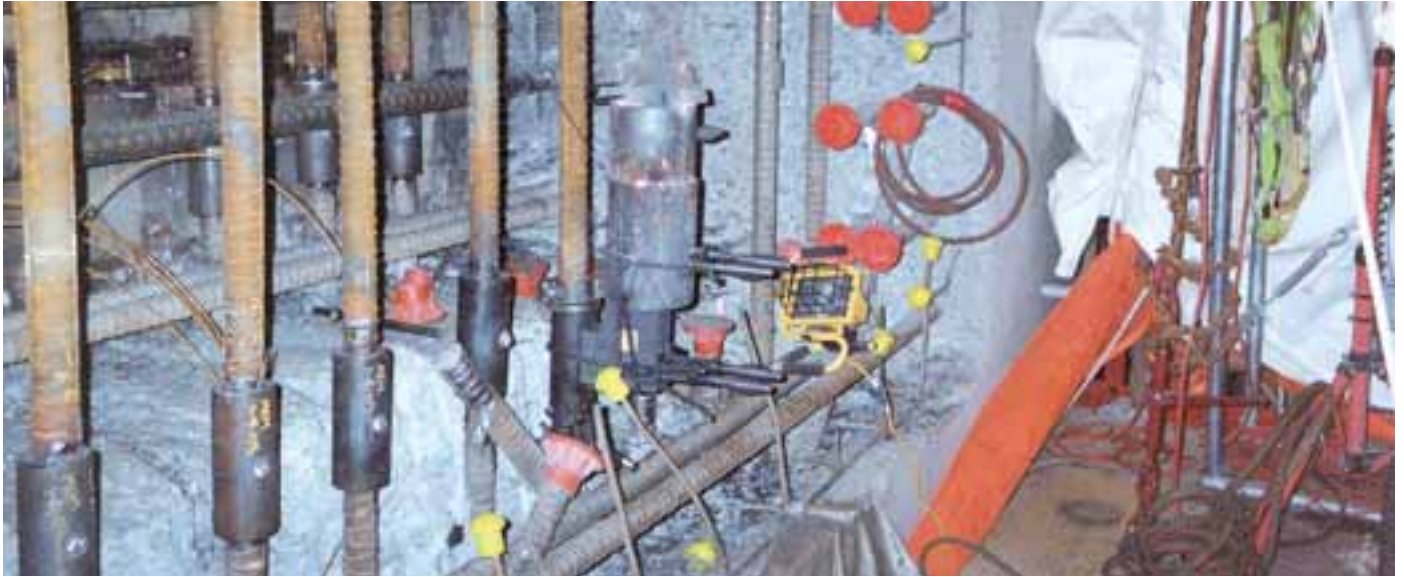
Repair Application - Nuclear Containment Structure
