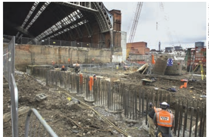
Piling work being completed outside of St. Pancras Station.
