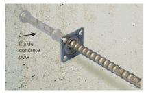
Screw in the taper threaded dowel bar and tighten with a pipe wrench.
