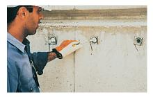
The form removal is quick and the protective metal disc is easily removed with a screwdriver.
