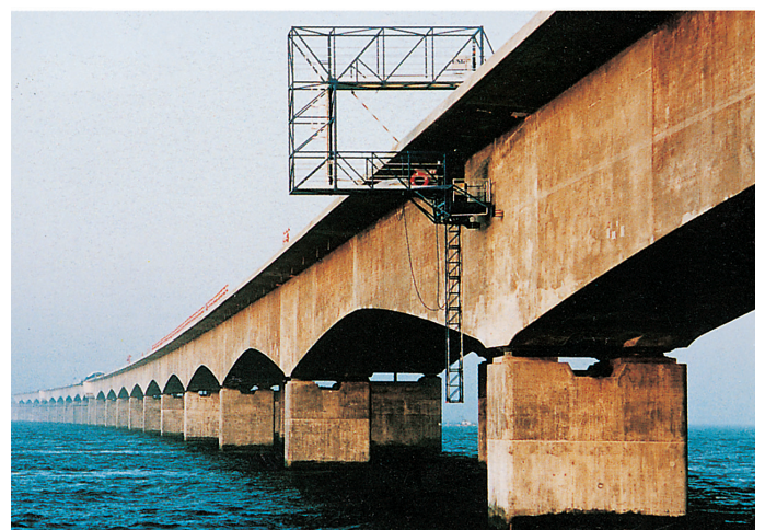
Storebaelt west bridge (DK)
