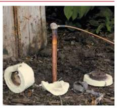
After one minute, break off the ceramic crucible. It can also be left in place, if desired.
