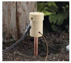
After preparing the ground rod and wire, position the Cadweld Plus One Shot and attach the lead to the control unit.
