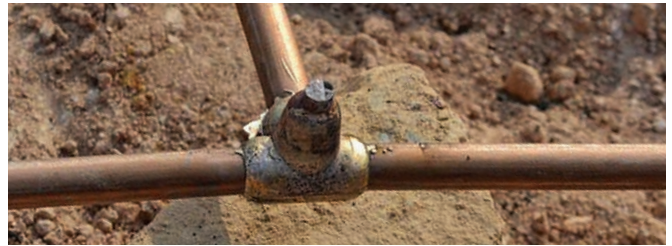
TA nVent ERICO Cadweld connection
