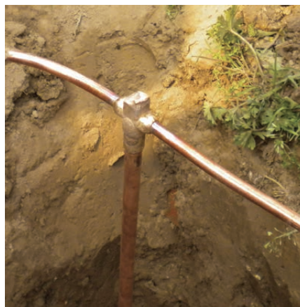
GT Cadweld connection
