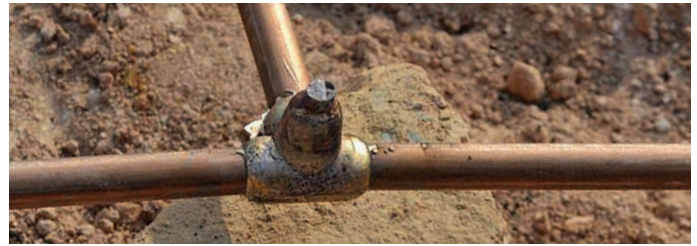
TA nVent ERICO Cadweld connection
