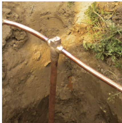
GT Cadweld connection
