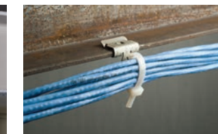
Cables from beam
