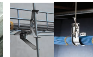
Cables from threaded rod
