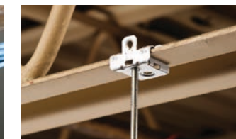
Threaded rod/chain/wire from beam
