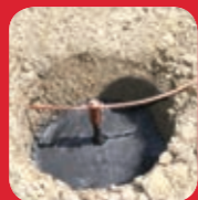
2. Ground enhancement material, GEM or Quickfill
