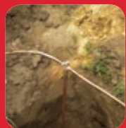
1. Copper bonded steel conductor, CBSC
