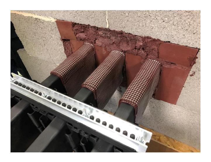
**nVent ERIFLEX FLEXBUS ADVANCED FIRE BARRIER** FIRE RESISTANT CONDUCTOR PENETRATION SEAL
