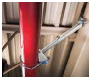
Lateral Telescoping Brace Assembly CSBTx – p. 31
