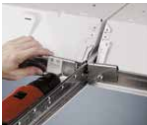
Seismic Lighting Fixture Clamp - p. 41
