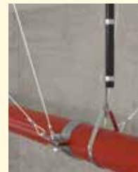
Pipe Rod Stiffener CSBRS1 – p. 36
