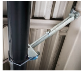
Lateral Telescoping Brace Assembly CSBTx – p. 19
